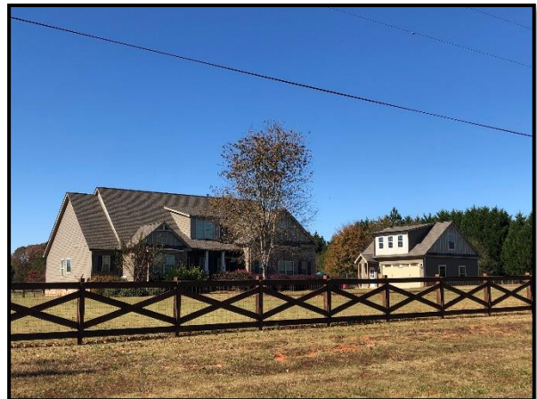
New Rural Residential Construction
